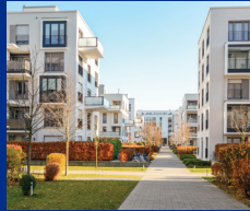
Maintenance and Remodeling
