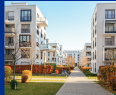
Maintenance and Remodeling
